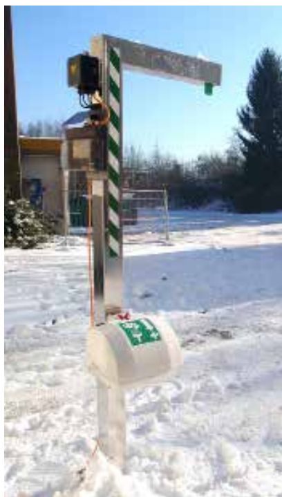
Nooddouche in wintermodus / Safety shower in wintertime
